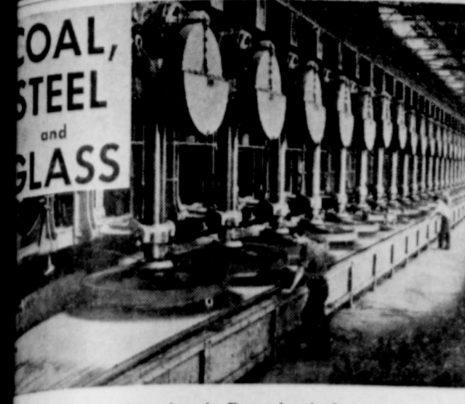
Polishing plate glass in Pennsylvania factory
