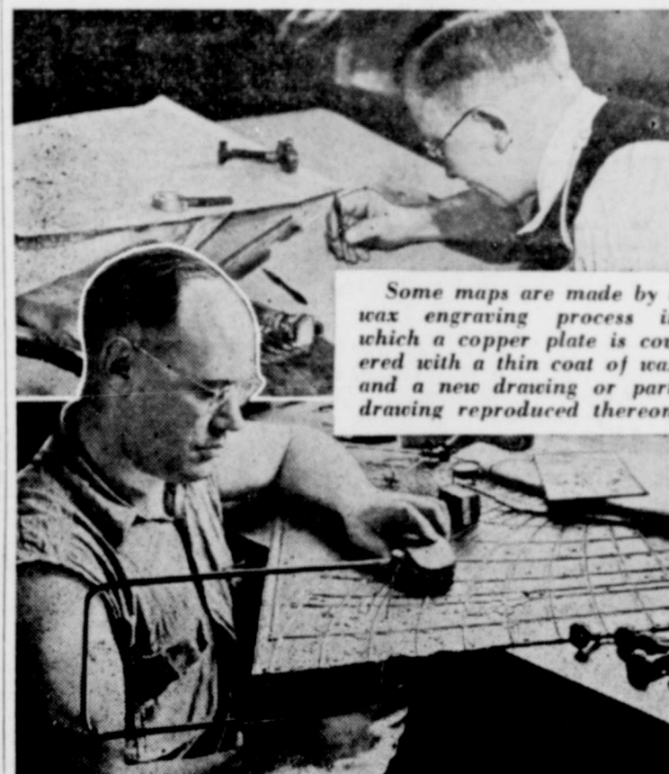
Where only a portion of the map is corrected, a "patch" is made by the wax engraving (electrotype) method and when completed is inserted into the existing map plate, thus bringing the map up to date. A foundryman is shown above sawing out a section of an original plate preliminary to such an insertion.
