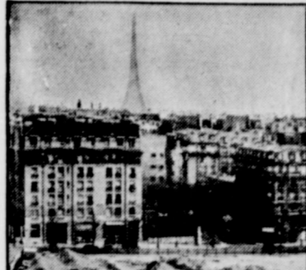
PARIS "CATA-COMBS" . . . Reproduction of maze-like catacombs under city of Rome is this scene in Paris, near Seine river, part of far-flung system of underground shelters under construction as protection against air raids in next war. Garden will be laid over trenches as camouflage.
