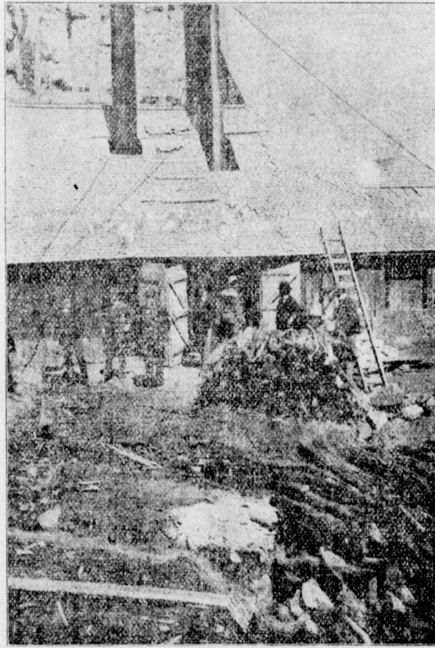
View of Stamp Mill, American Mine, Nogal, New Mexico.
