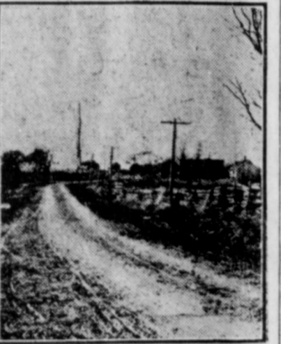
THE SAME ROAD MACADAMIZED.
