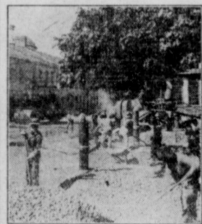
GETTING THE ROAD IN CONDITION. (From Good Roads Magazine, New York.)
