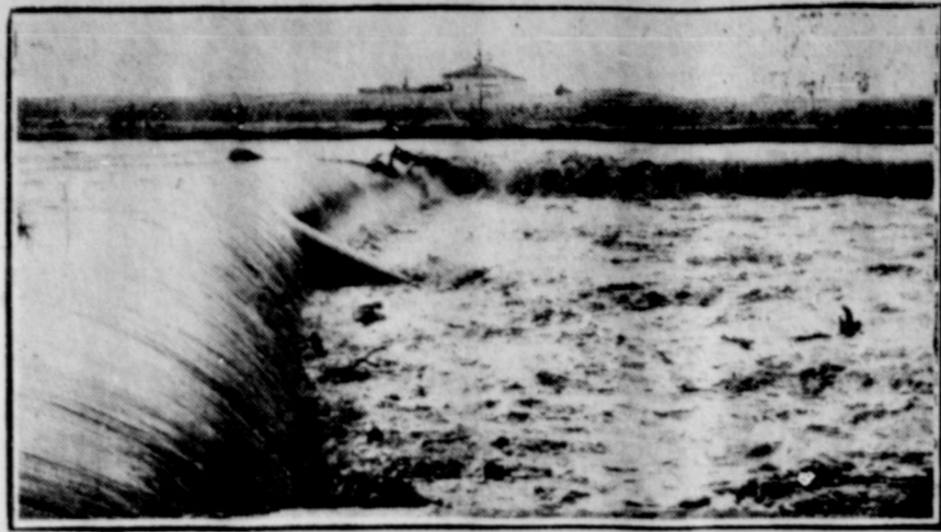
WATER WORKS DAM, SAN ANGELO, TEXAS.
