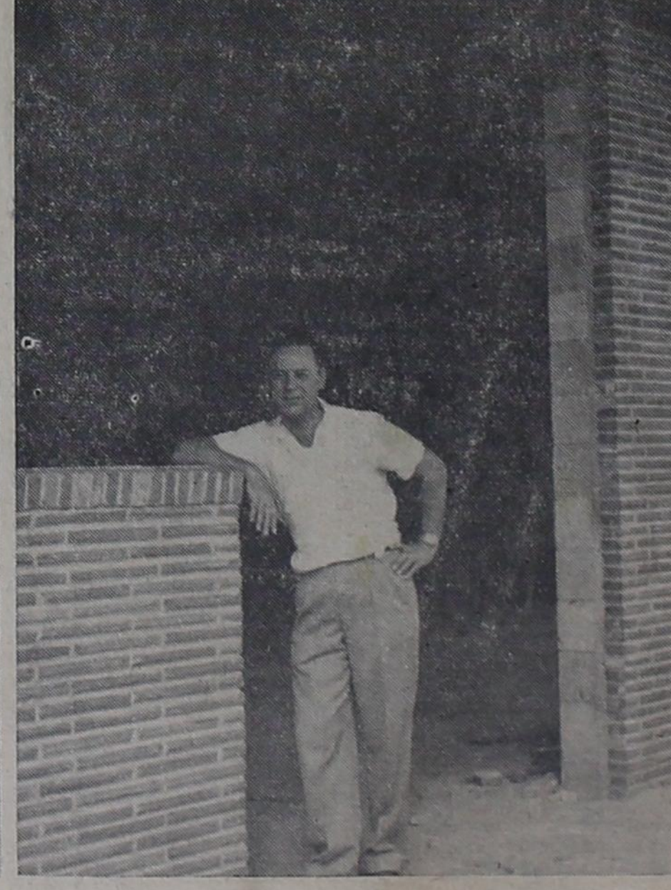
Through this doorway will walk our customers, the mamas of the greatest school kids on earth, says A. M. Wilson, as he poses in the doorway of his new super market which is now under construction. School is scheduled to begin before the contractor puts the finishing touch on the new building, but "we plan to be open sometime in September," Wilson says.
