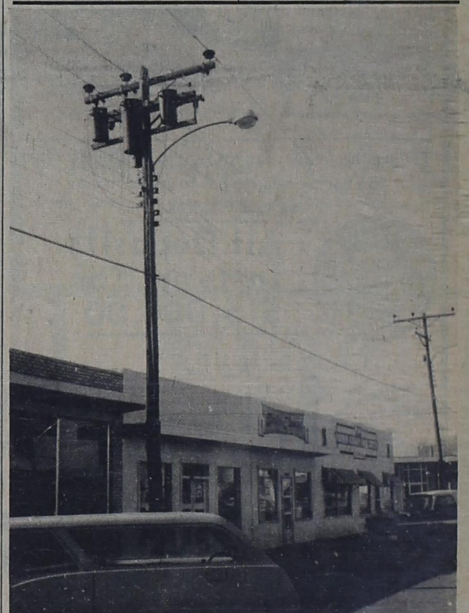
TO BE REMOVED -- Transformers, tall poles and numerous lines on Main Street from a half block northeast of Super Saweway through town is undergoing considerable change. Southwestern Public Service Company has been working on the lines the past few weeks and the results will be a neater appearance on Main Street.
