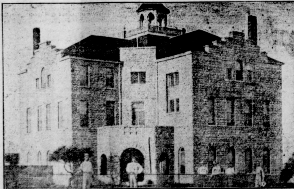
BRADY CENTRAL SCHOOL BUILDING.
