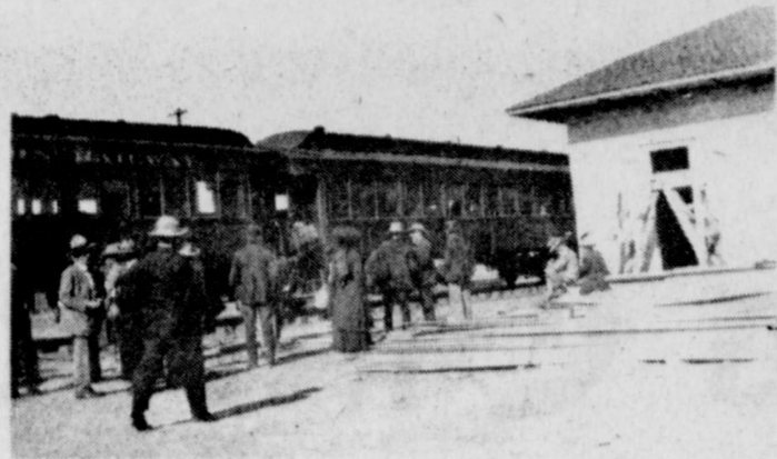
Picture No. 3 — Building the depot.
