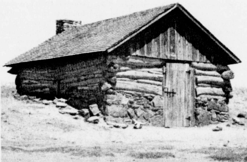
The Matador Half Dugout typical first home of a rancher on the plains
