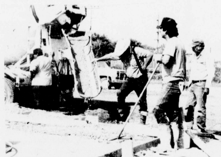
A crew supervised by Calvin "Jack" Jackson (in red suspenders) and Louis DeLaCruz (far right) pours concrete for the foundation for a new fellowship hall/kitchen/meeting room at Mt. Carmel Catholic Church last Thursday. The building will be a prefabricated metal building with a large meeting room and kitchen facilities located just to the south of the church.
