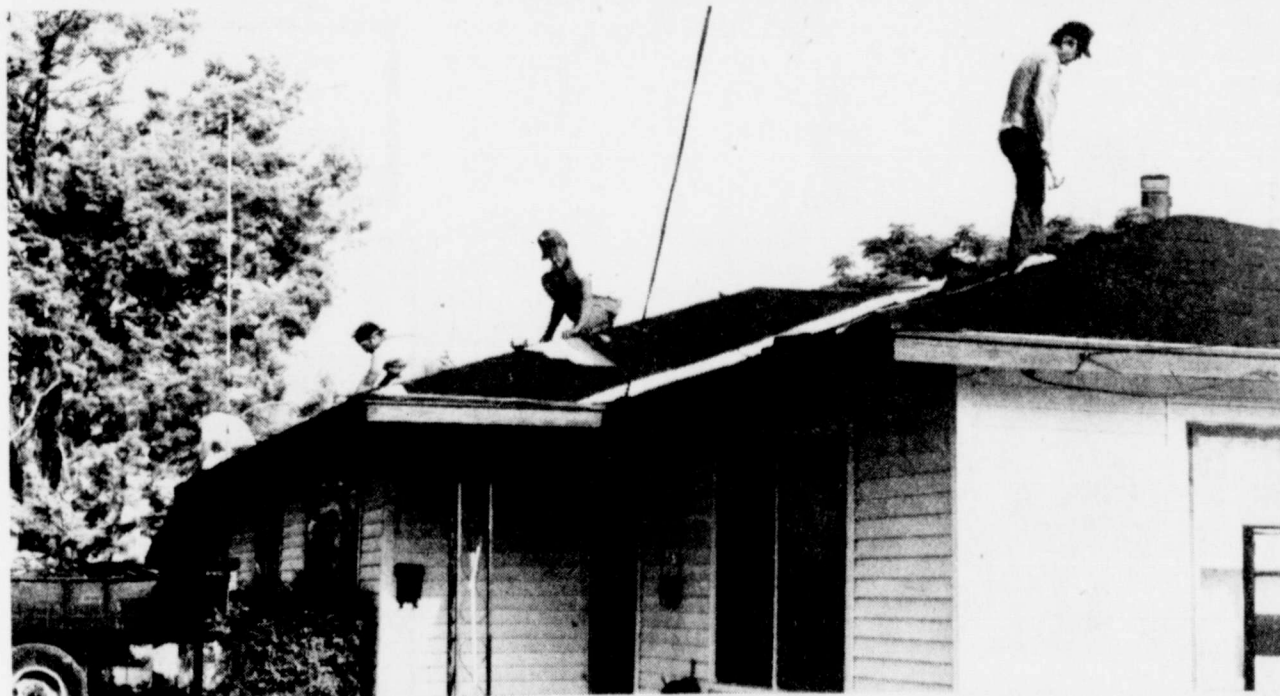
Pictured above are a few of those who helped with re-roofing the James Powers house the first of this week. Mr. Powers, a teacher in the Winters Independent School District, suffered a severe heart attack as he began the project last week. From left to right are Russell Stewart, Robert Cook, Lucius Wood, and Robert Russell.
