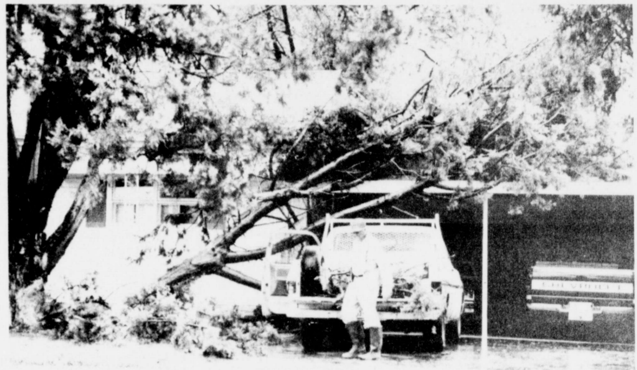
Martin Middlebrook surveys damage caused when a large cedar branch fell on his house.
