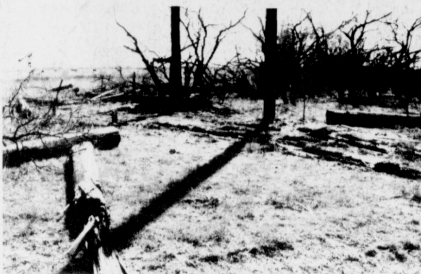
Splintered poles are evidence of lightning damage done to a large power transformer north of Winters.
