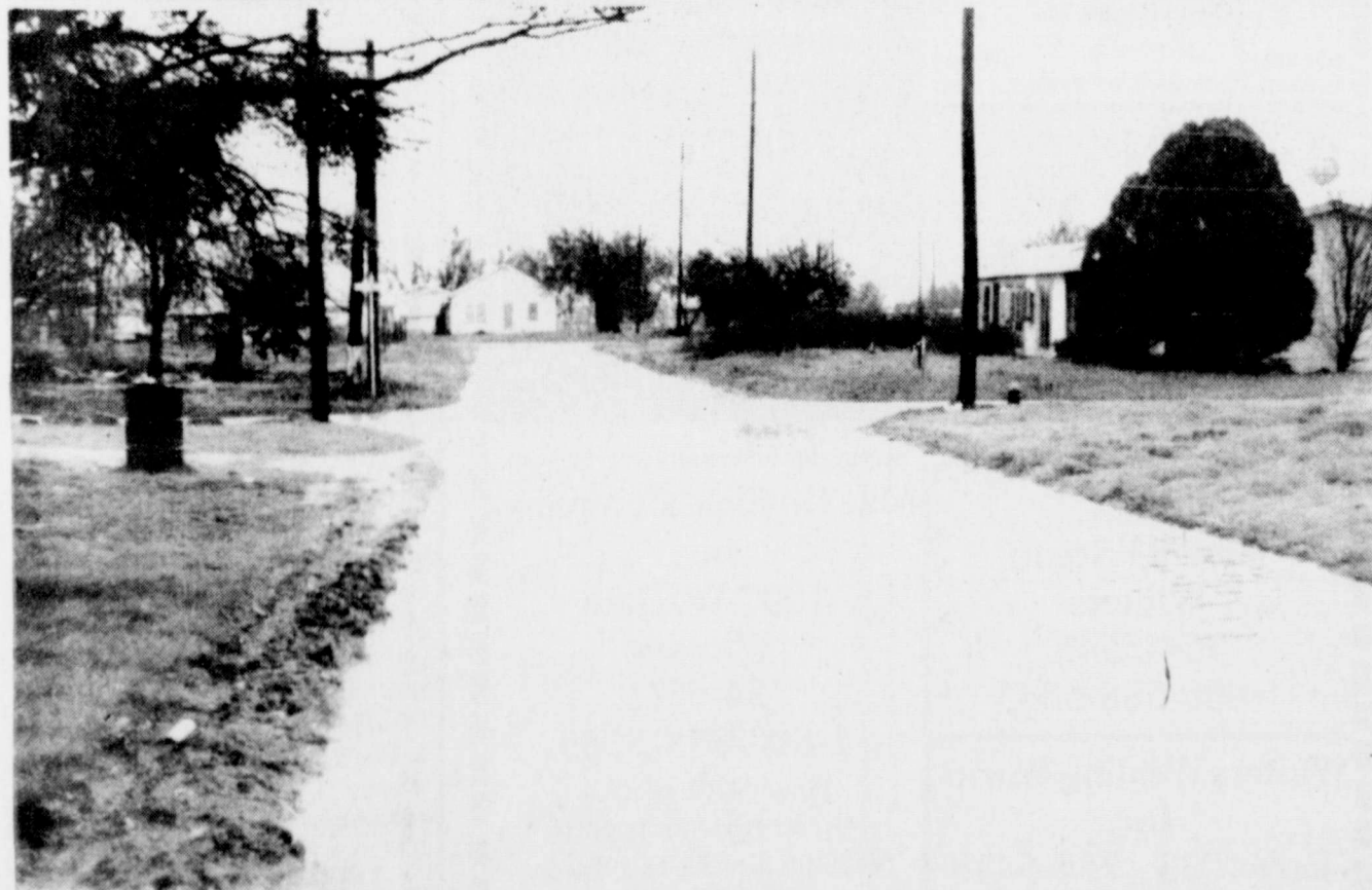
WATER, WATER EVERYWHERE — This scene at Fannin and Parsonage streets was a familiar sight all over Winters as heavy rains fell Monday, Monday night and Tuesday. Continued rain has plagued the Winters area causing pot holes on city streets which maintenance crews have not been able to repair because of the unseasonably wet weather.
