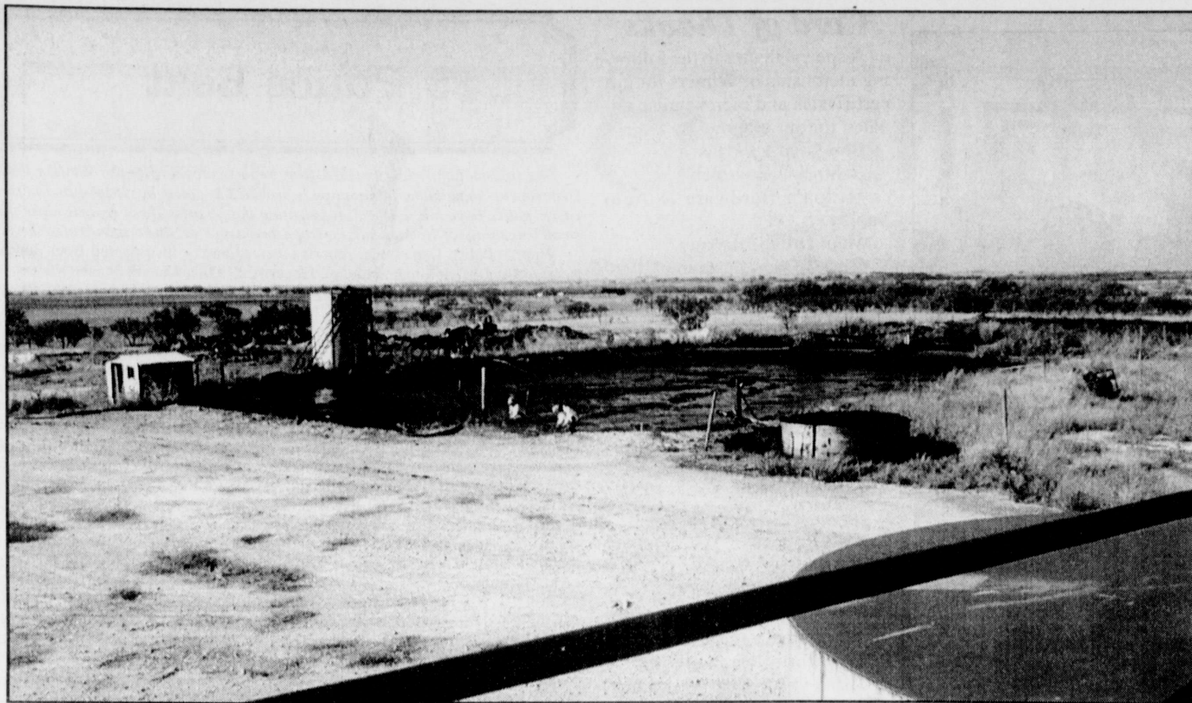
AN ABANDONED COMMERCIAL SALTWATER DISPOSAL facility located just west of Poe's Corner on SR 384, was the site of a $403,017 clean-up effort by the Railroad Commission of Texas—the largest saltwater disposal clean-up in the state's history. The site consisted of 4 large pits and 11 tanks containing basic sediment and water, crude oil, and saline produced water. This picture was taken in early October as contractors began the remediation process.
