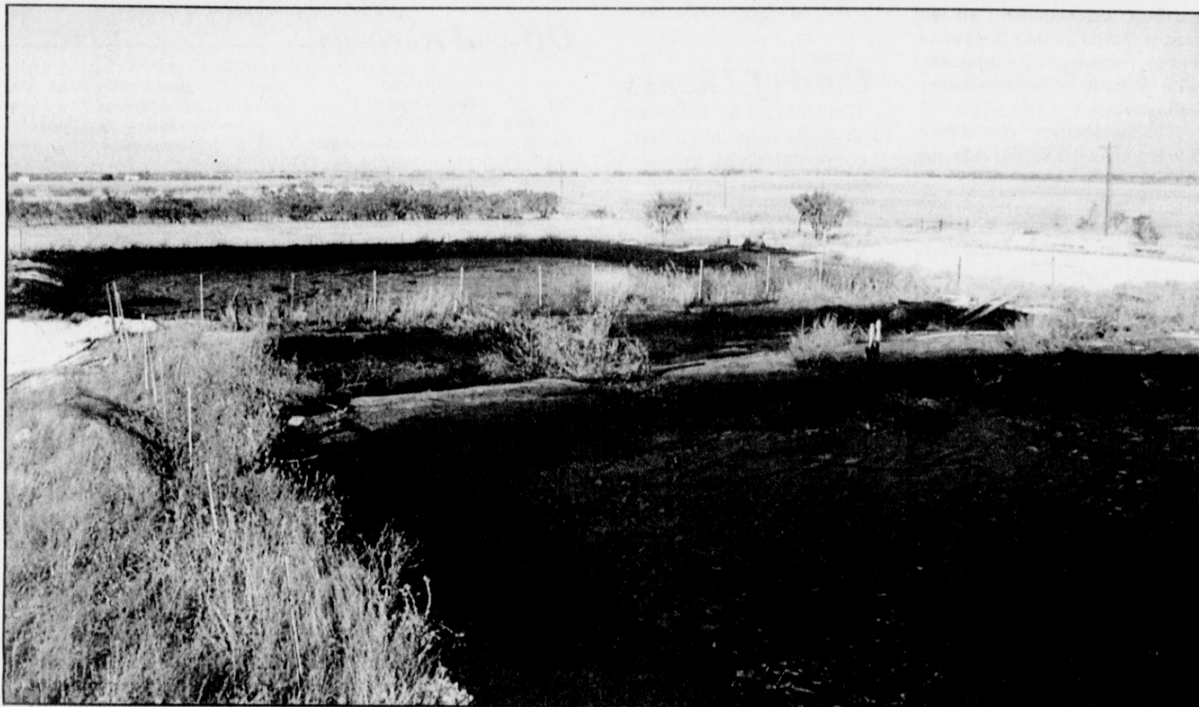
THE RUNNELS COUNTY SWD, INC. was the site of a major clean-up effort by the RRC to remove 22,285 barrels of basic sediment, crude oil, and saltwater, which was hauled to Borden County Waste Disposal in Gale. The remediation also disposed of 680 cubic yards of crude oil contaminated soil. BS was vacuumed from these pits, liners removed, and soil tested for contamination. The six acres are now ready for grazing according to the Commission.
