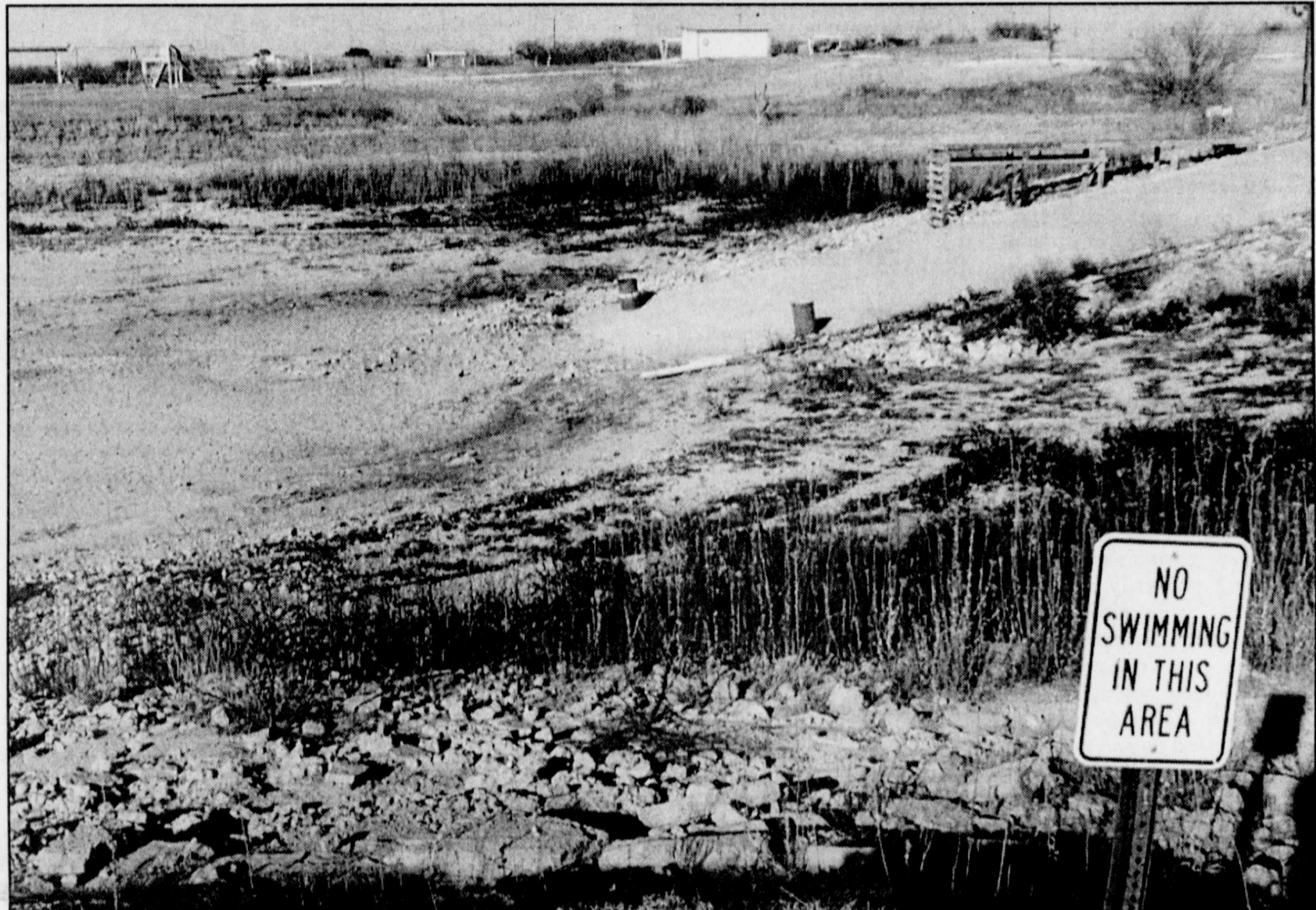
WITH THE WATER LEVEL at 20-22 feet below normal, Elm Creek Reservoir has only approximately 20 months' supply of water, according to City Water Superintendent Jack Davis, Jr. Steps are being taken to pump water from Old Lake Winters and private wells into the Reservoir. At top right is the dock and boat ramp which is now approximately 75 yards from the water's edge.
