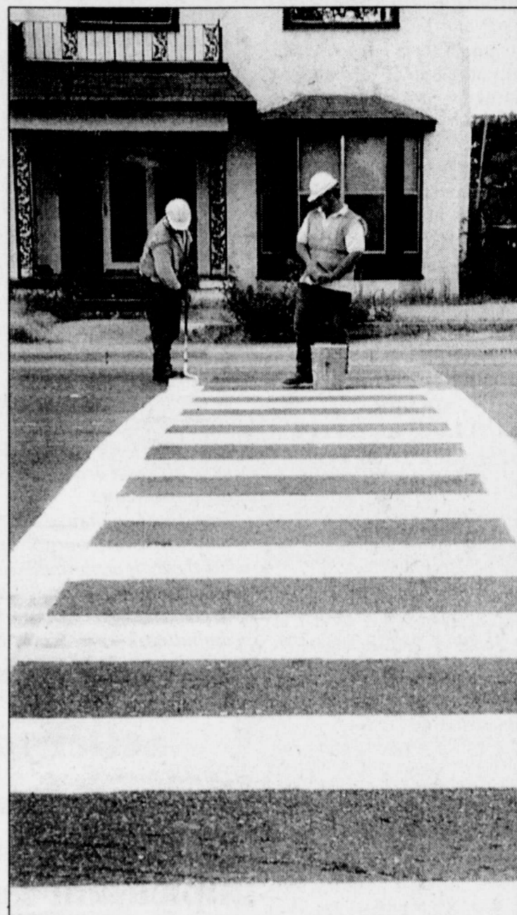
A NEW COAT OF PAINT is applied to the school crosswalk at Main and Jones by workers with the Texas Highway Department. Classes at WISD start Monday, August 13, and drivers are urged to use caution and observe the reduced speed limits around the school area.
