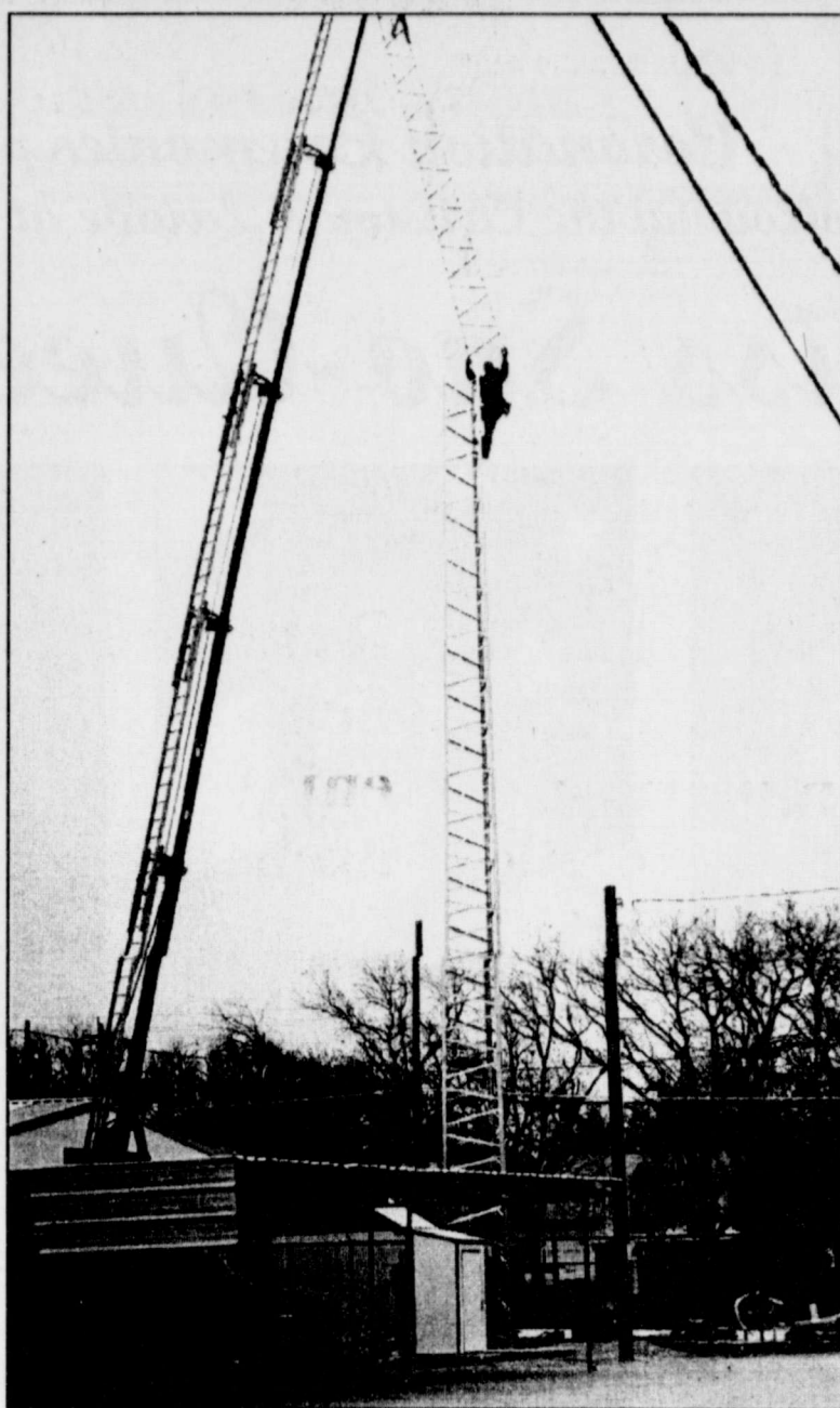
QUITE A HIGHWIRE ACT took place recently, by Butch Strickland, at 131-A N. Main, behind Potbellies Restaurant. This 100 ft. tower was installed by Texas Communications.
