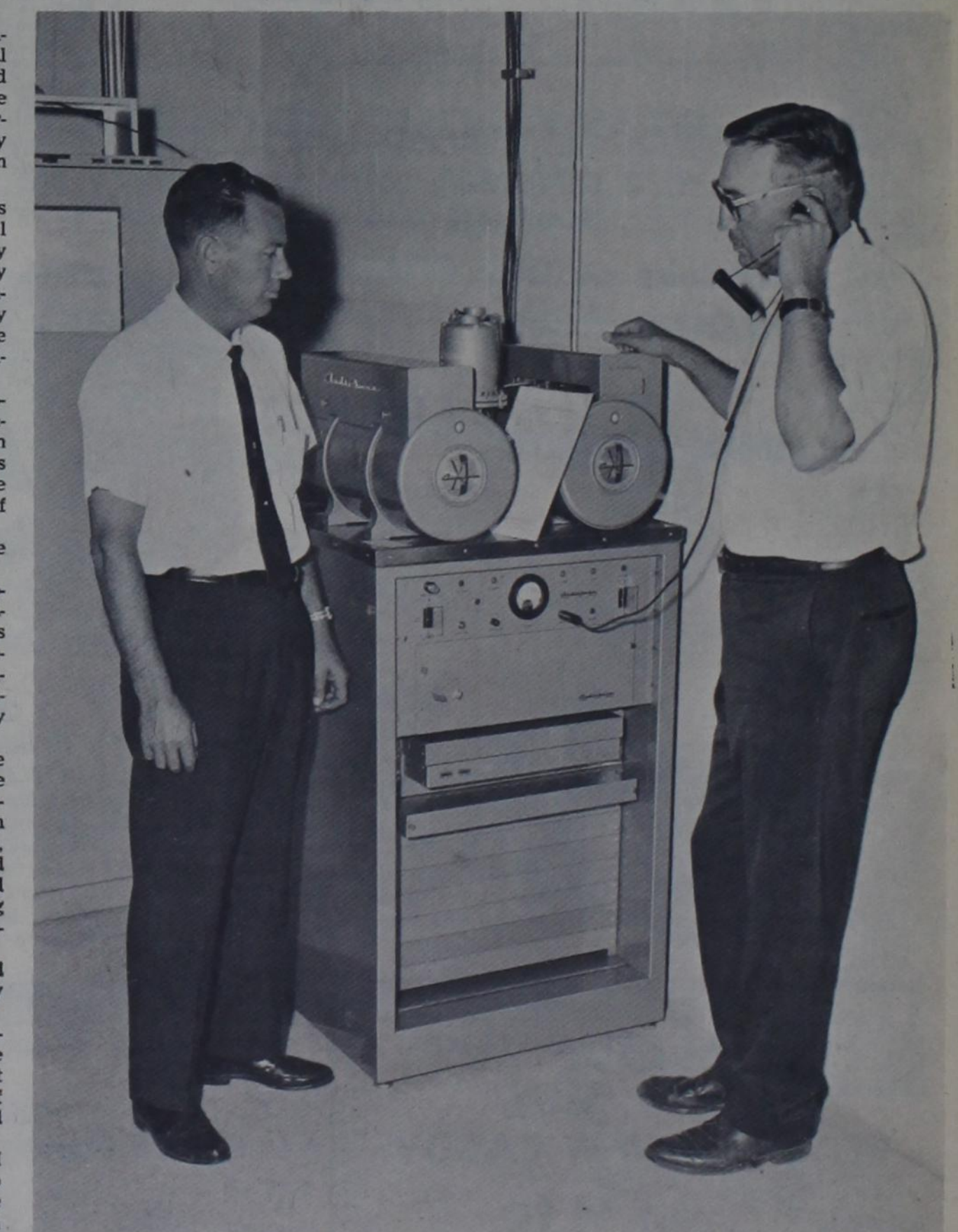
BILL WOODARD , left, manager of West Texas Telephone Company, is shown with Ed McLeRoy, agricultural representative and vice president of the First State Bank, as they examine the new time and temperature equipment installed recently in the telephone building. Correct time and temperature is available at any time by dialing 647-3133.
