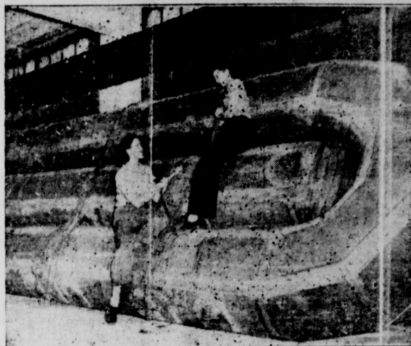
Massive rubberized cotton pontoons like the one above aid in giving added mobility and striking power to U. S. armored forces. By the use of such pontoons with heavy steel treadways, new armored force bridges can be erected faster and carry heavier loads than any other military bridge in existence.
