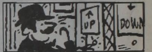
The first successful electric elevator was installed in New York City in 1889.
