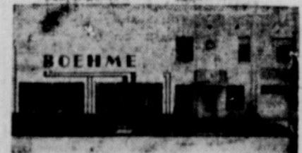
Our New Plant, Built in 1941
