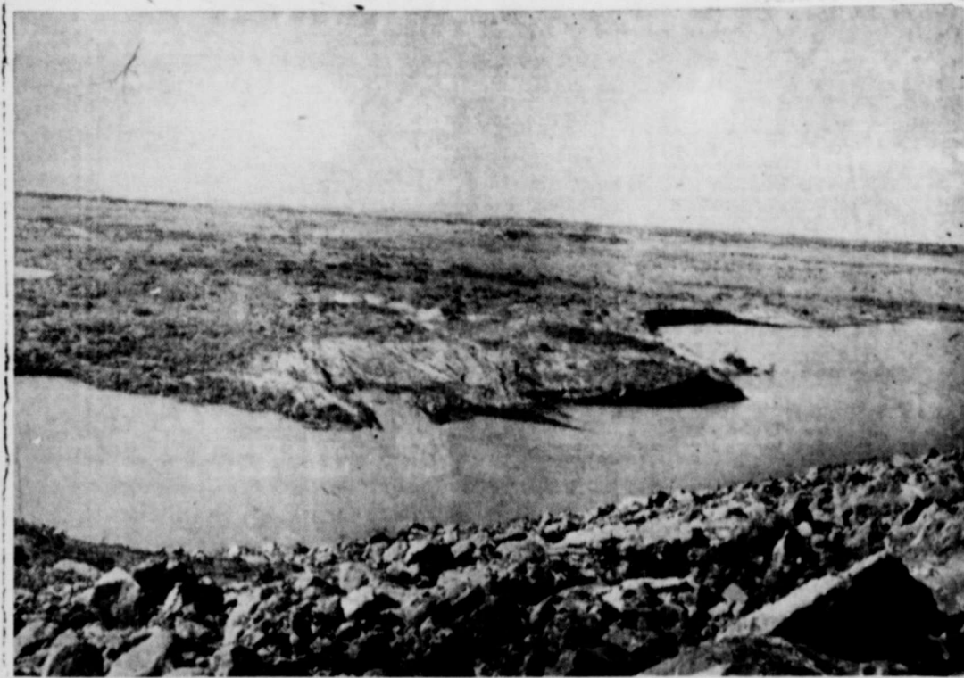
OAK CREEK LAKE'S FIRST WATER—This picture, taken from atop the last section of Oak Creek Dam, now being closed, shows the first water to be impounded by the dam to give Bronte and Sweetwater a municipal water supply. At this point Kaiser Creek and Oak Creek meet in a "V" formation immediately above the dam. Deepest spot in the water shown is between 20 and 30 feet.
