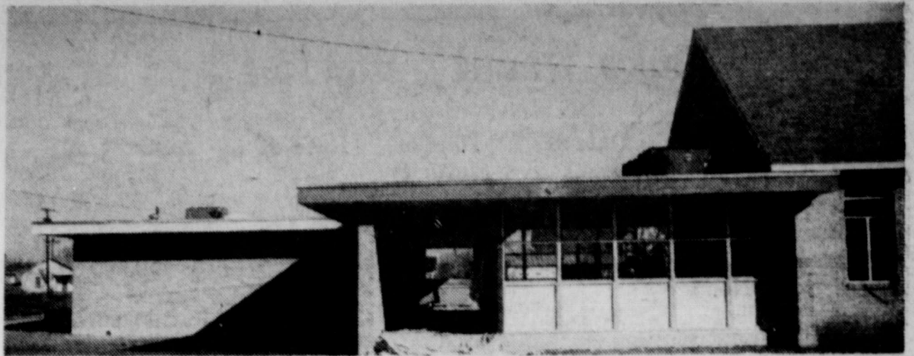
View of New Methodist Church Building from South
