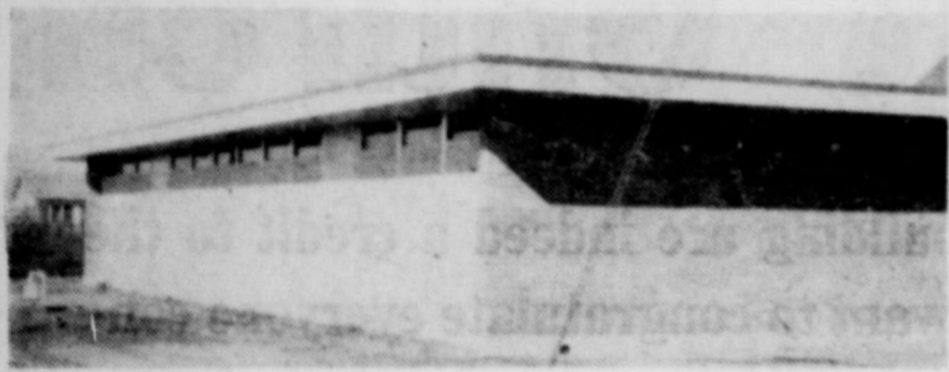
FROM THE REAR —Here is a rear view of the Sunday school wing. This shot, taken from the south, shows the full length of the new wing.
