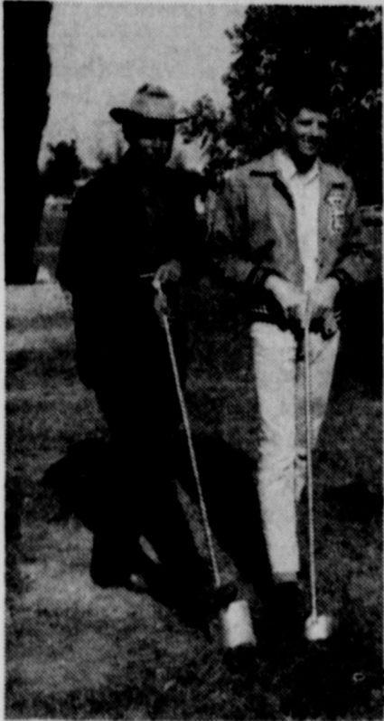
ONE OF THE FIRST — The ground breaking ceremony on Nov. 18 initiating construction of the new agriculture building for Bronte High School featured one ground-breaker who was a member of the first vocational agriculture class of Bronte High School. Board member Jacob B. Morrow was a member of the original class, and is shown here with Davis Corley, present FFA president.
