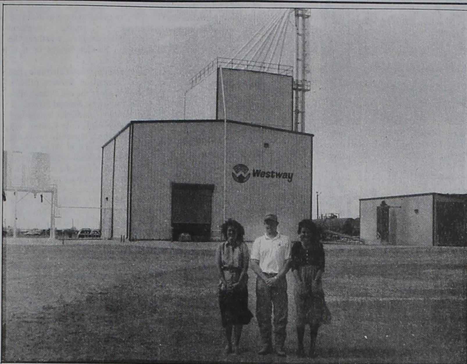
WESTWAY TRADING CORP. will hold a ribbon cutting today (Thursday) at 10 a.m. for the expansion at their Dimmitt facility. Shown are company personnel (from left) Denise Schilling, administrative assistant; David Darnell, terminal manager of
