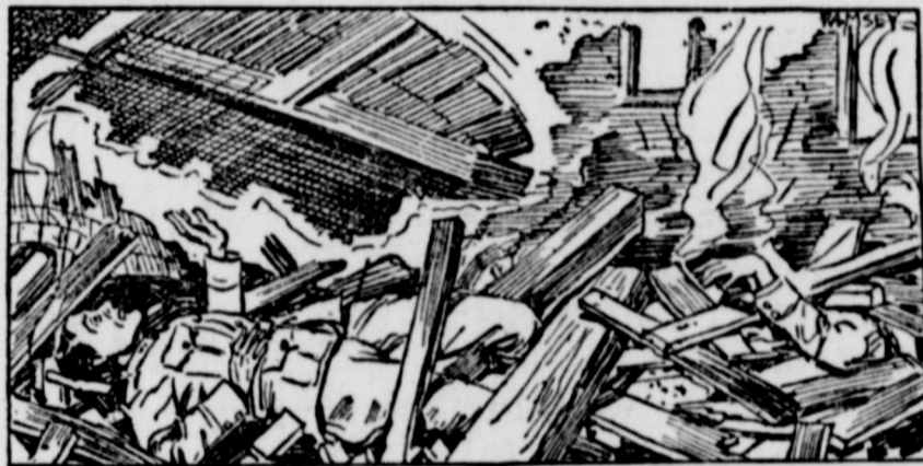
Bill's Legs Were Pinned Between Two Beams.
