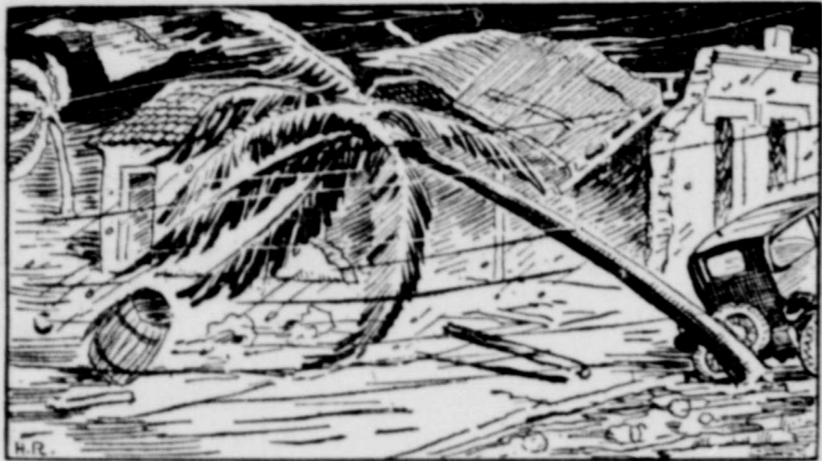
Roofs Went Flying Off Houses.
