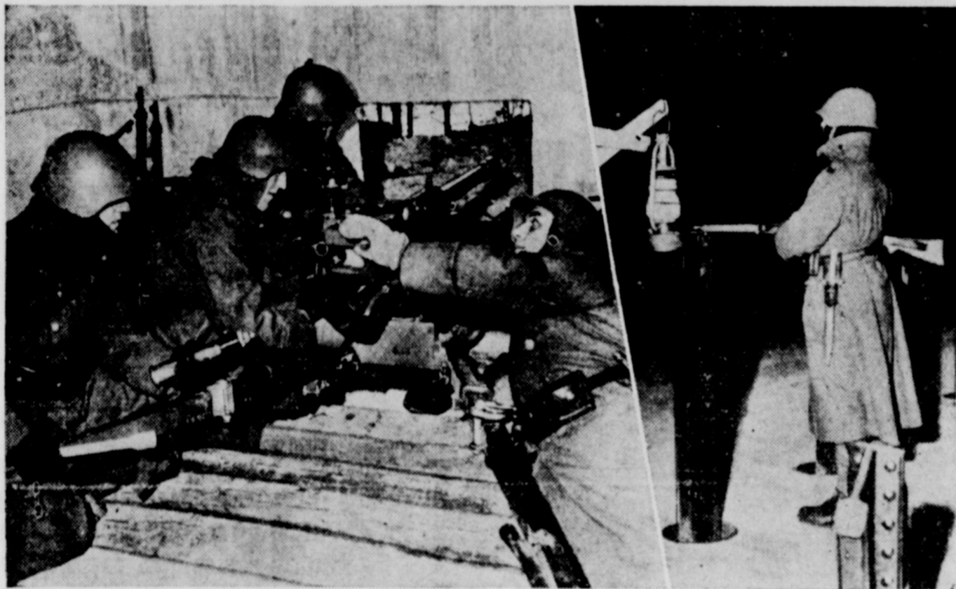
A Swiss anti-tank squad is pictured (left) on a small but well-protected link in its "William Tell line." Practically every border village of Switzerland has several of these fortifications. Right: Everlasting vigil is maintained in danger zones. These iron sticks are a formidable barrier erected against tanks of a belligerent mechanized force. Switzerland's army consists of 600,000 well-trained, well-equipped men.
