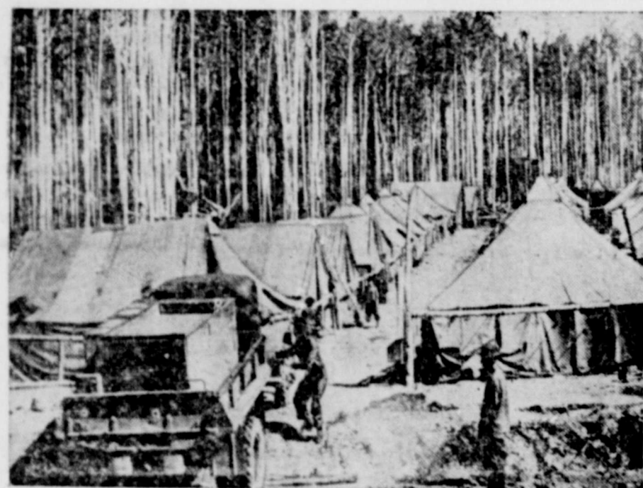
Contractors camp along the Alaskan highway job. Camps are so located that the thick poplar growth serves as protection against winter storms. The camp area is graded to assure proper drainage.
