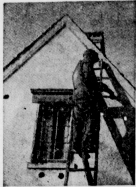
Insulating homes, as shown here, is another important fuel conservation order. It will reduce fuel consumption from 10 to 20 per cent.
