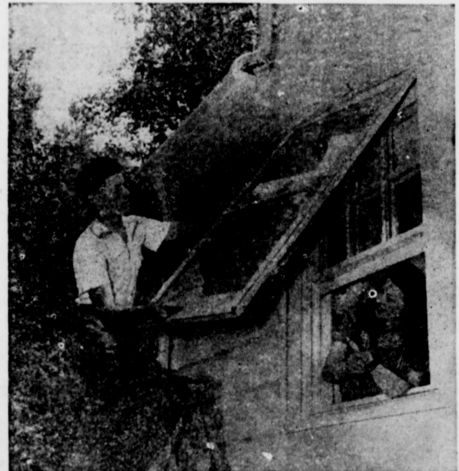
Heading the list of the ten commandments for fuel saving, as mentioned in this article, is window conditioning or fitting storm sashes. This, too, will save on the winter's fuel bill.
