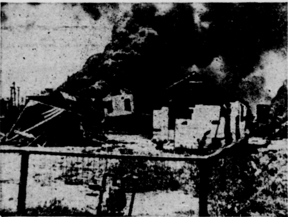
MANY LEFT HOMELESS IN TEXAS CITY . . . When fire and explosion wrecked industrial district of Texas City, on Galveston bay, Tex., even many persons who escaped death or injury were left homeless. Miles away windows were blown in, brick walls crumbled and many persons were injured or killed by flying debris. It may be weeks before the total casualty or property loss will be known. First reports, placing the injured and dead at several thousands, have been largely confirmed.
