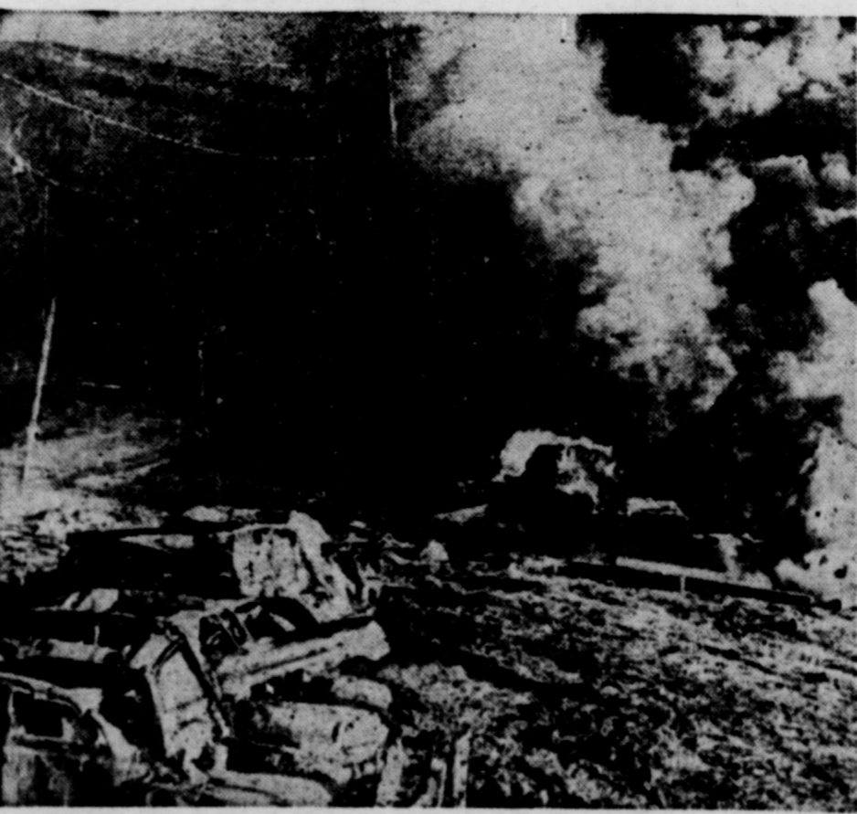
NEW FIRES, EXPLOSIONS ADD TO HAVOC . . . With new fires and explosions adding to the carnage of the Texas City, Tex., tremendous explosion, early reports proved to fall far short of final damages to this industrial city, located on Galveston bay. Photo shows later blazes in the waterfront area. With the leveled Monsanto chemical plant in the background, wrecked cars, all blasted in the original explosion, are shown in the water-soaked area as agencies of cities, states and federal government sought to bring relief.
