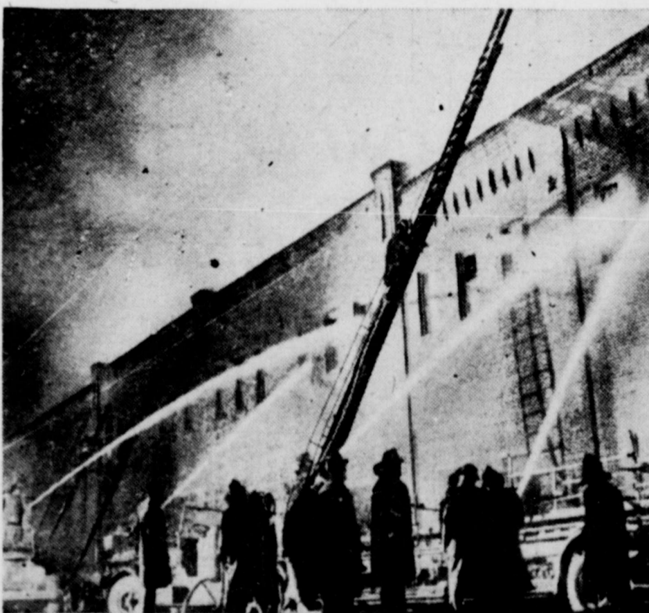
SUGAR GOES UP IN SMOKE . . . The sugar shortage wasn't helped a bit by this raging fire which swept warehouses of the American Sugar Refining company plant in the shadow of the Williamsburg bridge on the Brooklyn waterfront. Ten firemen were overcome or injured in the five-alarm blaze, and tons of water were poured on to the flames, which threw great billows of smoke high into the air and burned for hours.
