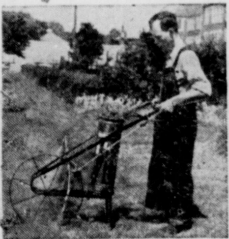
Sprayer mounted on cultivator as designed by Michigan State college.
