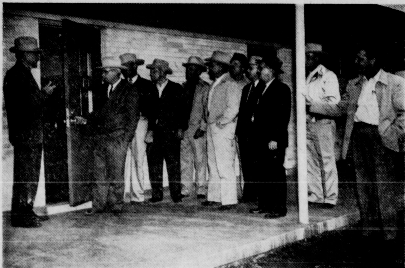
LET'S LOOK INSIDE—Contractor Houston Hill opens a classroom door so school trustees can take a look inside. Left to right are F. M. Johnson, inspector, Mr. Hill, Wilson Bryan, Jack Cowley, Bryan Gartman, Bob Godwin, J. I. (Dusty) Rhodes, construction foreman, Architect Ed. Wilson and his assistant, Joe Cunningham, J. C. Harwell and T. R. McAden. The latter had a sub-contract for heating and plumbing.
