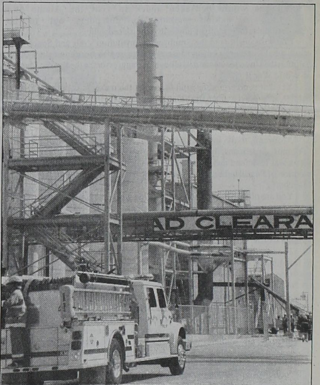
FIREFIGHTERS STAND BY AT AMERICAN MAIZE-PRODUCTS —Dimmitt volunteer firefighters stood by Tuesday afternoon after a flash in a smokestack at American Maize-Products in Dimmitt. The fire produced dark smoke for a few seconds, but the brief problem was quickly corrected. Photo by John Brooks
