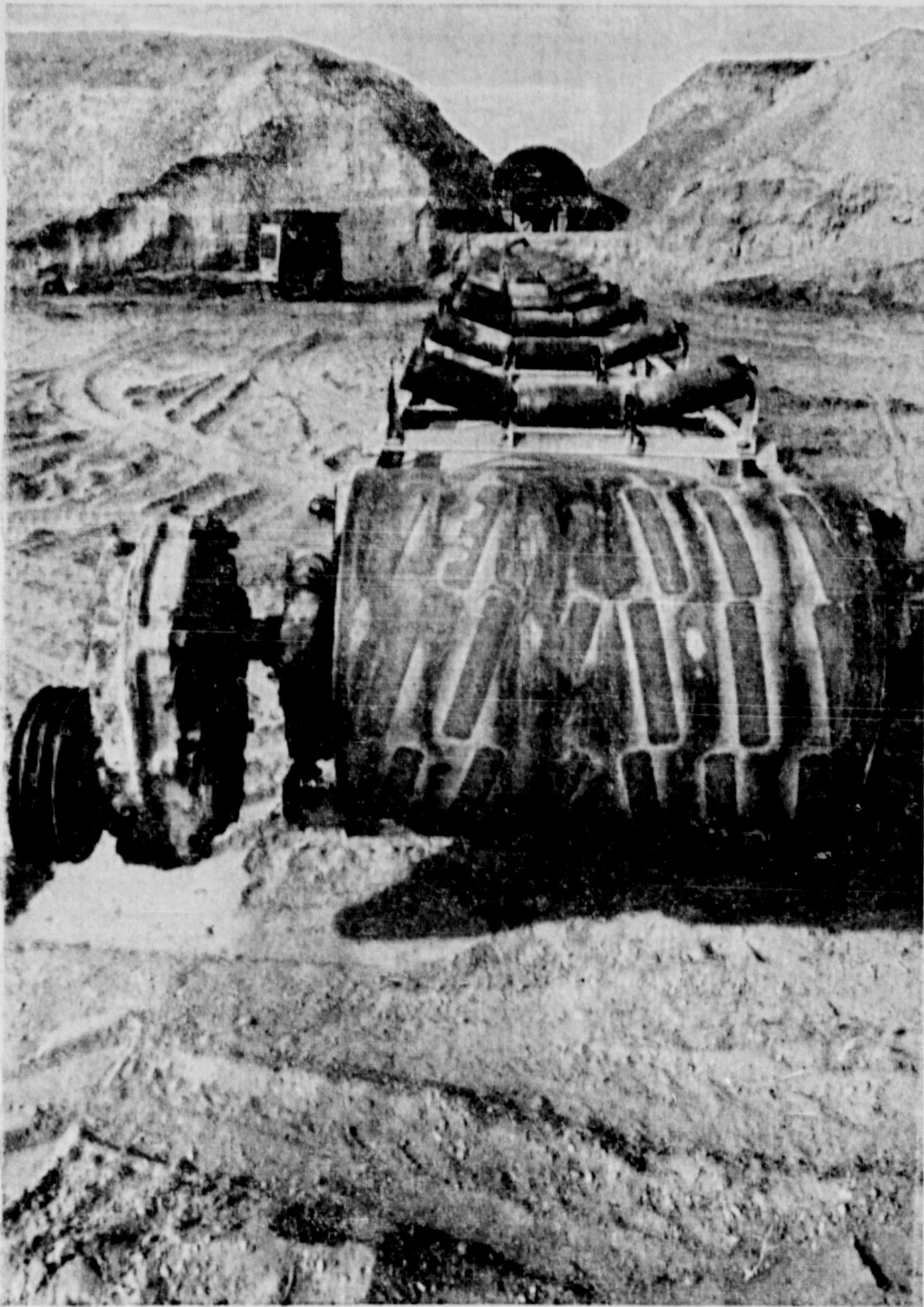
Conveyor for Giant Grinder at Dam
