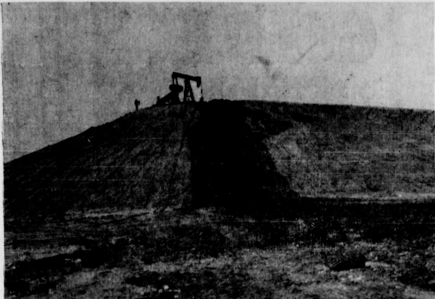
Oil Field Mounds Have Raised Pumps Above Water Level
