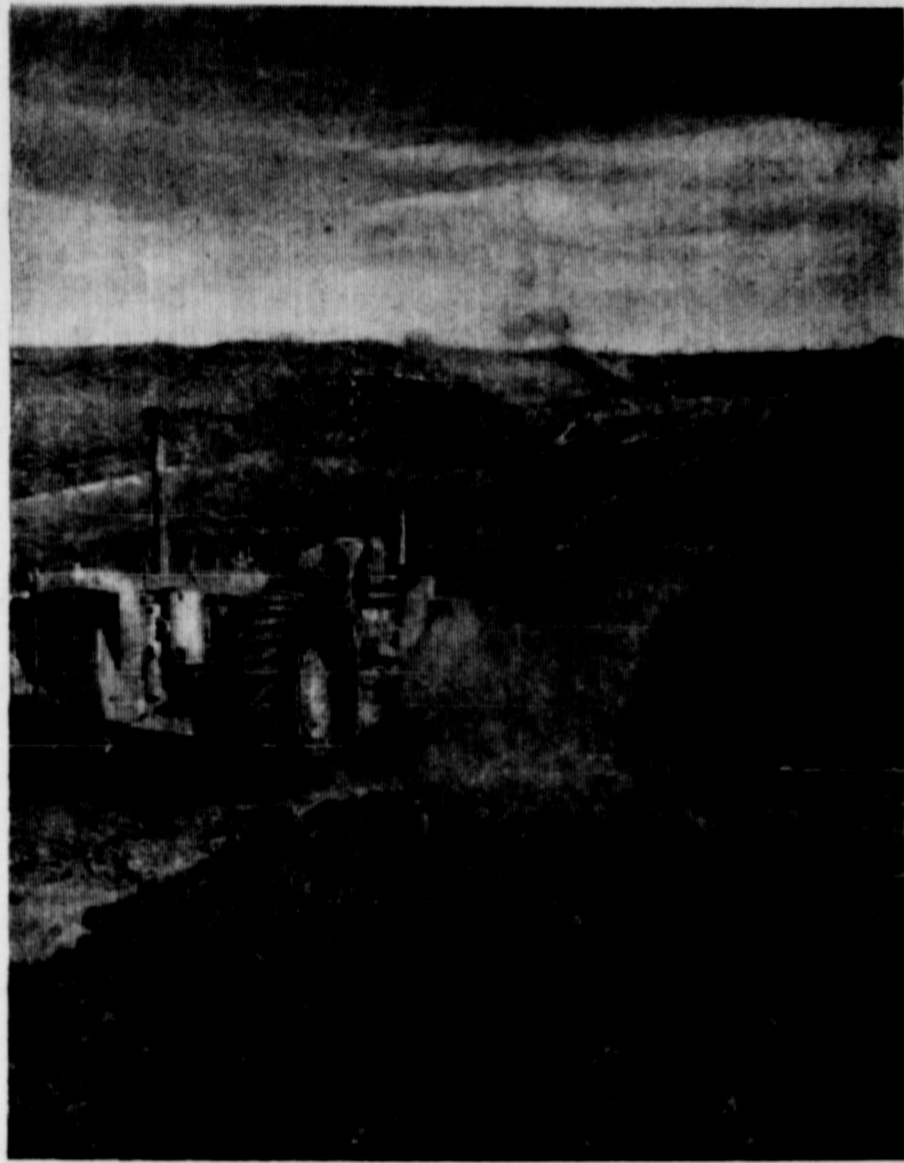
Big Machines Clear Out An Area
