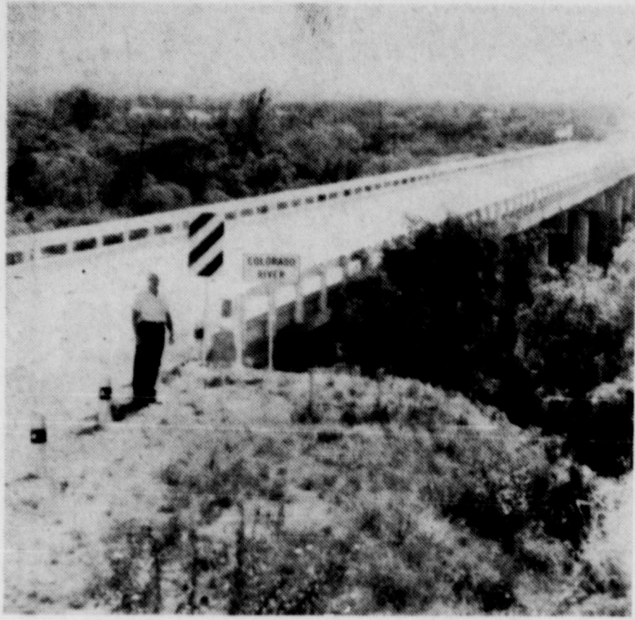
NOW UNDERWATER — The bridge across the river on the road to Sterling City used to look like this. The past few weeks, however, have seen wa-
