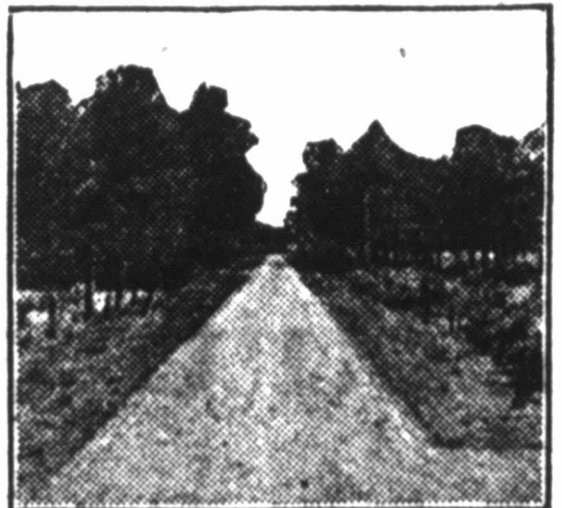
Permanent Road in Connecticut.
