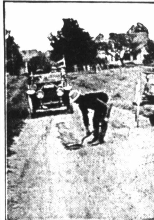
Patrolman Patching State Road.
