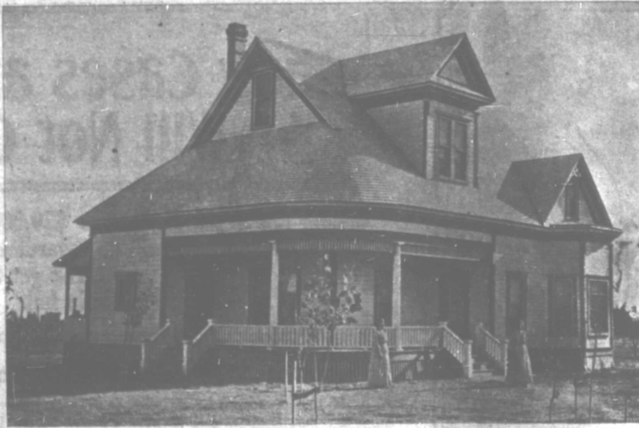
Residence of A. A. Williams, Portales, New Mexico.
