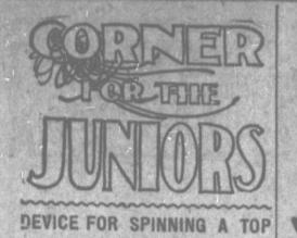
"Y" Shaped Wire Frame Holds Spike of Toy Until Sufficient Momentum Is Acquired.
