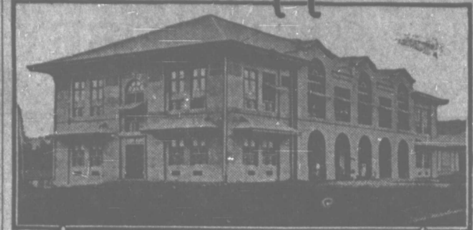
HIGH SCHOOL BUILDING, Cebu
