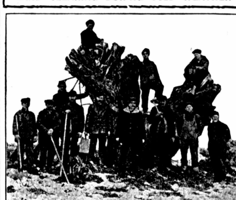
Blasting Stumps in Winter With Low Freezing Explosives.
