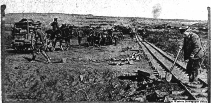
The reconstruction period is now sweeping over all of the battle-scarred area of France and the roads are being rebuilt. This photograph shows a scene on a road in the vicinity of Cambrai that was mined by the retreating Germans. The British constructed a light railway and a new road.
