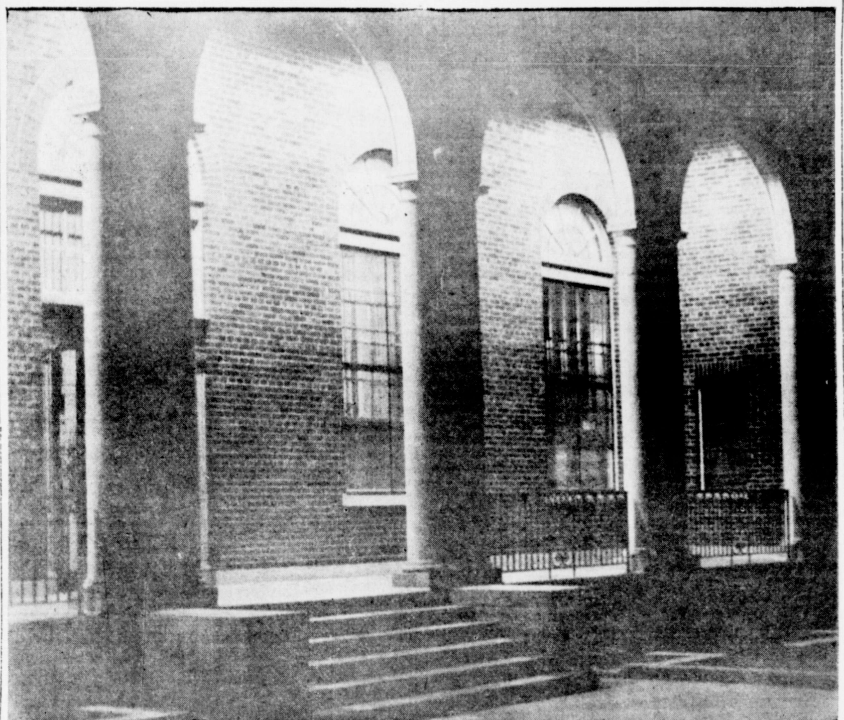
The warm glow of evening shadows, expressing at once dignity and an invitation. Up these steps pass more of Cisco's people than go through most any other portal. This engraving, etched in the plant of the Cisco Daily Press was made from a night photograph made by Bill Morton of the Mills-Morton studio.
