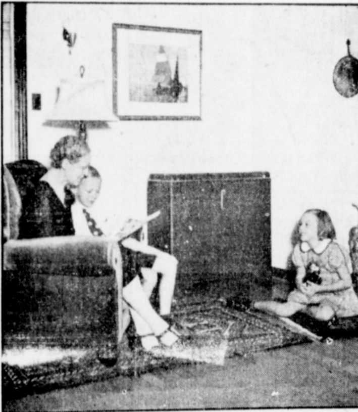
This sample photo shows a vented circulating gas heater in the home of one of our customers.
