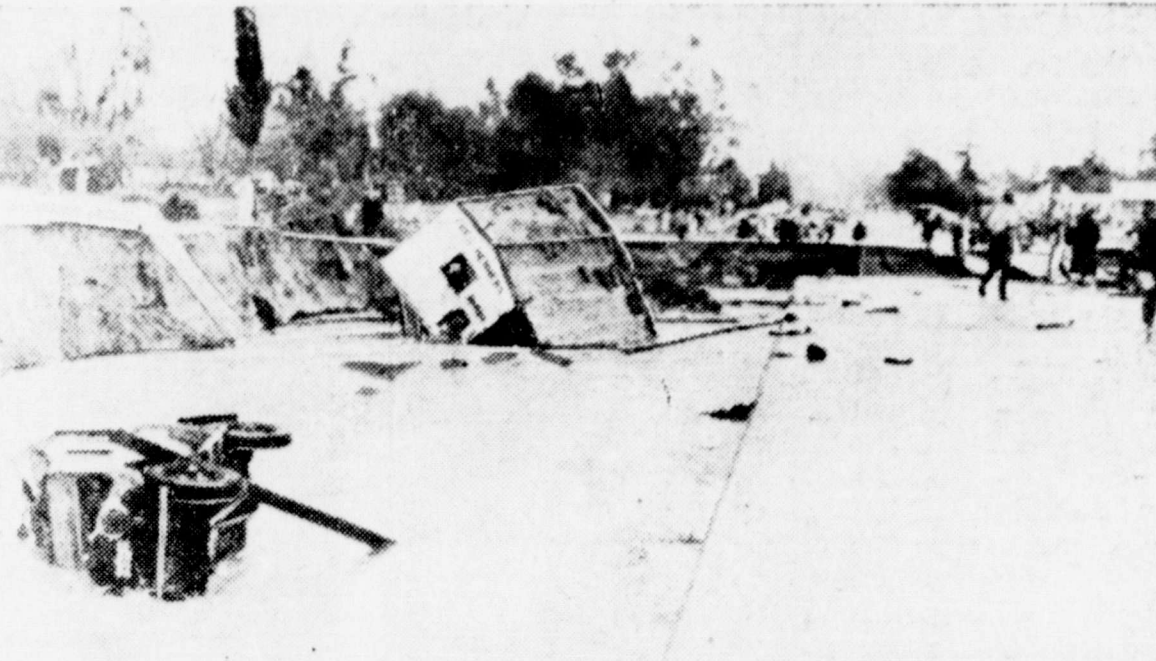
A little thing like a concrete street meant nothing to the torrents that rampaged through the Los Angeles area after four days' downpour. This picture, taken in the suburb of Burbank, shows pavement washed out by the fury of the flood. Note the shack and car overturned at the side of the street. This was just a small part of the tremendous damage wrought by the floods that inundated 30,000 square miles of southern California and ravaged more than 100 towns.
